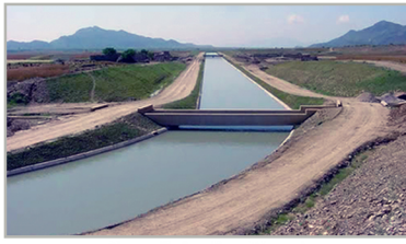
Open Irrigation Canals
